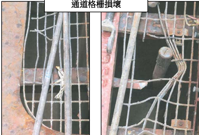
Badly wasted floor plate (thinned and holed) 通道地板嚴重鏽蝕 (變薄及穿孔)
