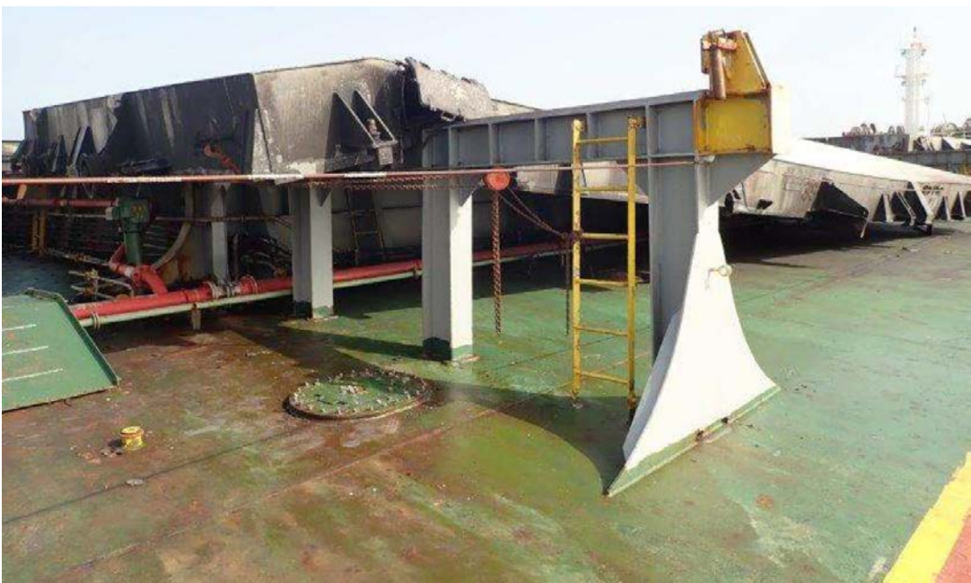
Figure 5 Aft end of No.3 C/H hatch cover starboard panel
