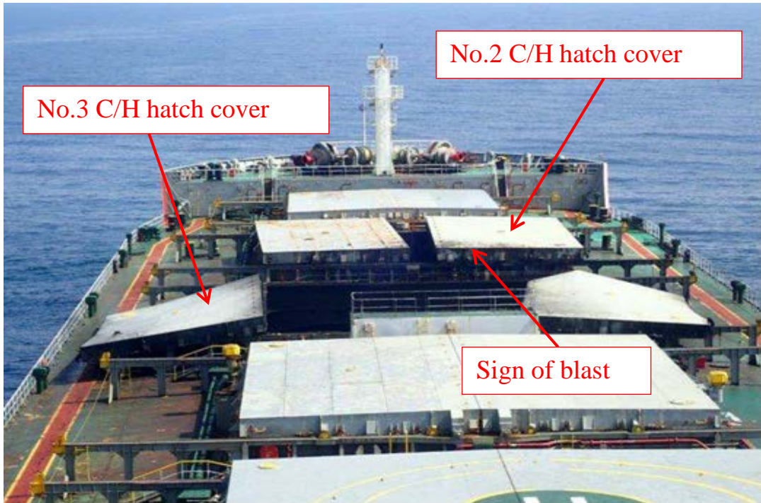
Figure 2 The dislocated No.2 and No.3 C/Hs hatch cover panels (looking forward)
