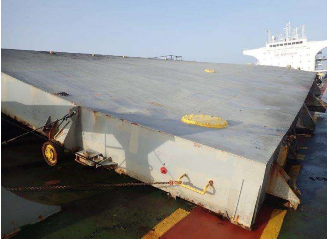
Figure 6 Forward end of No.3 C/H hatch cover port panel
