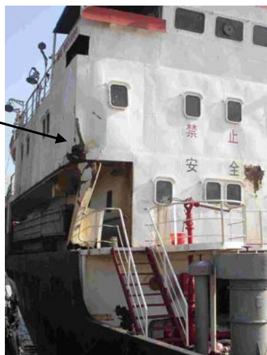
Fig. 10: Damage on Crew Accommodation of Vessel Caused by Collision
