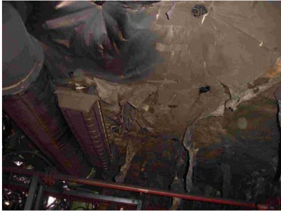
Fig. 21: Ceiling of Fire Station
