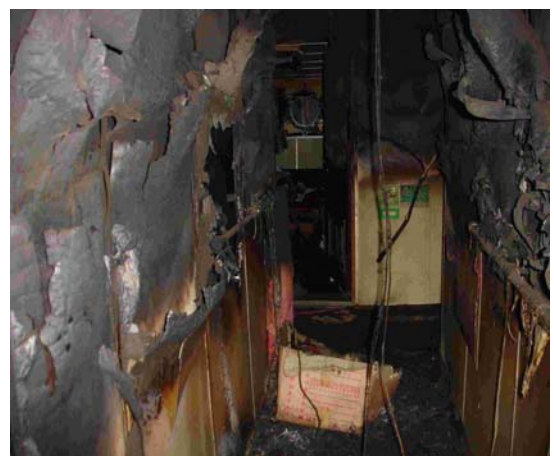
Fig. 20: Corridor behind Fire Station
