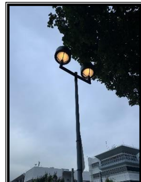
Streetlamp Luminaire glowed with PV LED Units at Dusk
