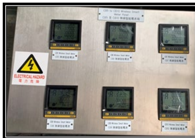
Six Meters to monitor power consumption
