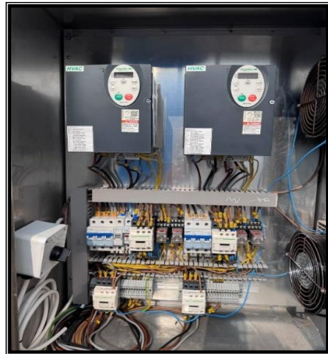
Newly Installed Control Panel for VSD Units
