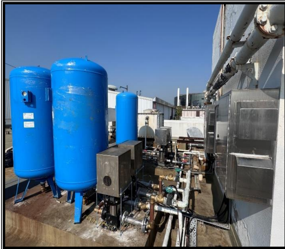
Newly installed fresh and flush water pump set with VSD Technology for Optimising Energy Efficiency
