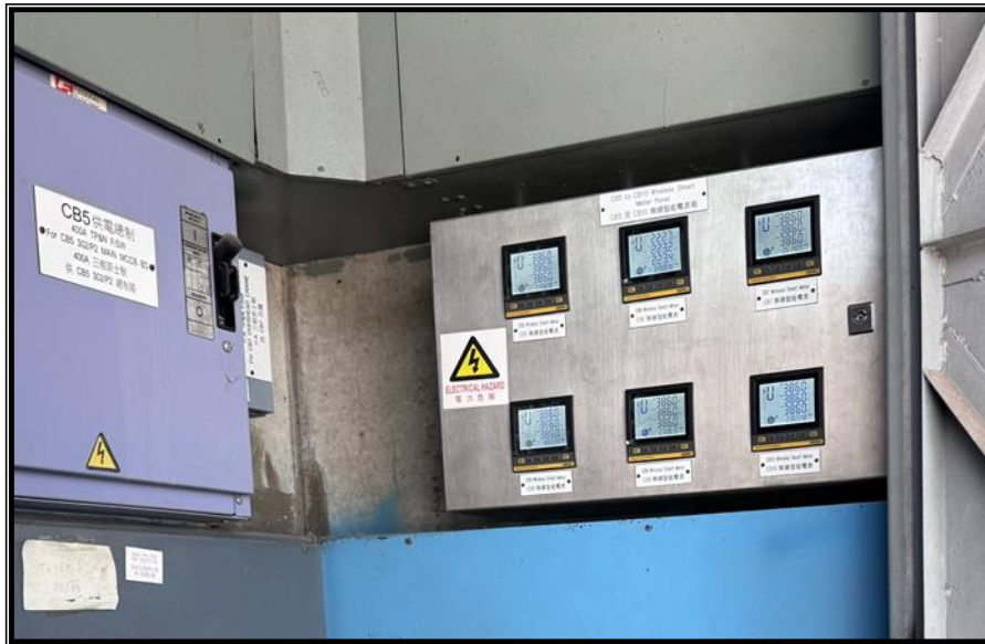
Six Smart Meters for monitoring power consumption
