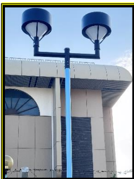
A Streetlamp Pole replaced with PV LED Units
