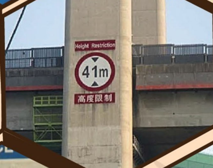
汲水門大橋區域 Kap Shui Mun Bridge Area
