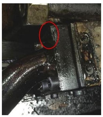
Numerous foam application nozzles throughout the engine room that were closed by hardened foam creating the potential for the failure of the fire fighting system
