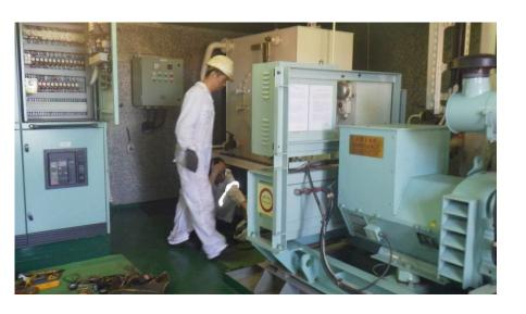
During a PSC inspection a blackout sequence test will be conducted. This will simulate a blackout of the main power and test the emergency generator's ability to supply emergency systems. Emergency generators are becoming an issue. Typically, vessels are detained as they can be started but do not go on load automatically.
