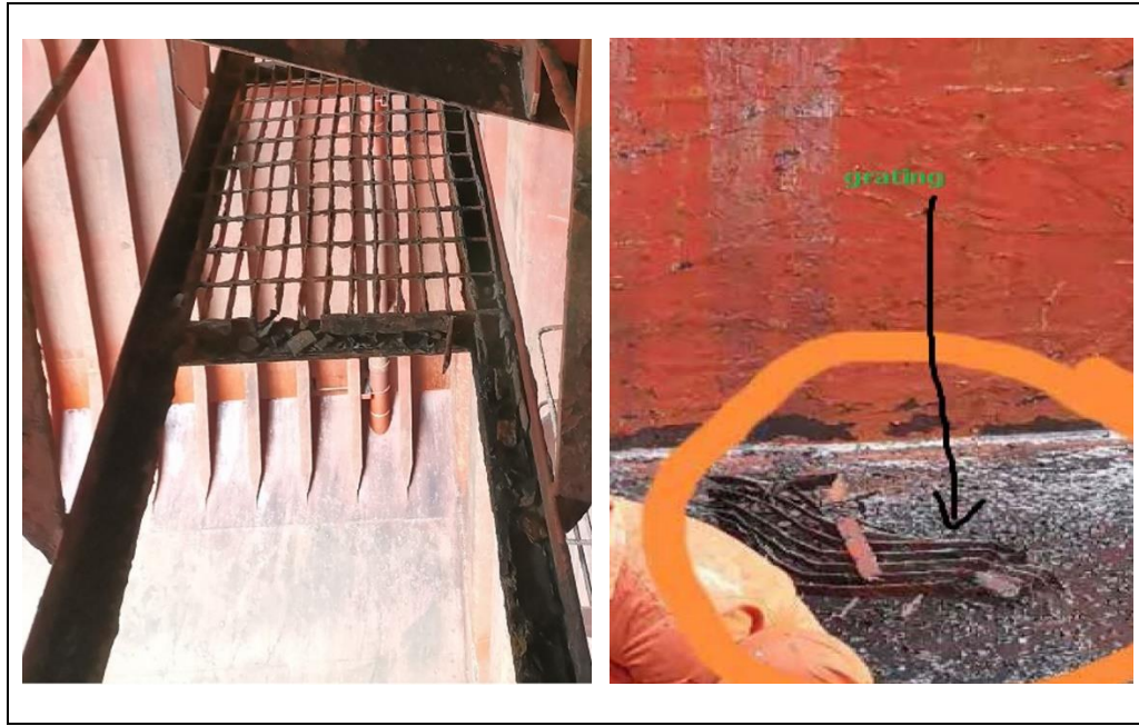
Figure 5: The condition of the detached grating and its support frame
