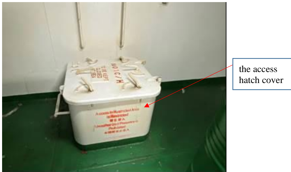
Figure 5 The access hatch of the No.1 cargo hold was located in the windlass control room
