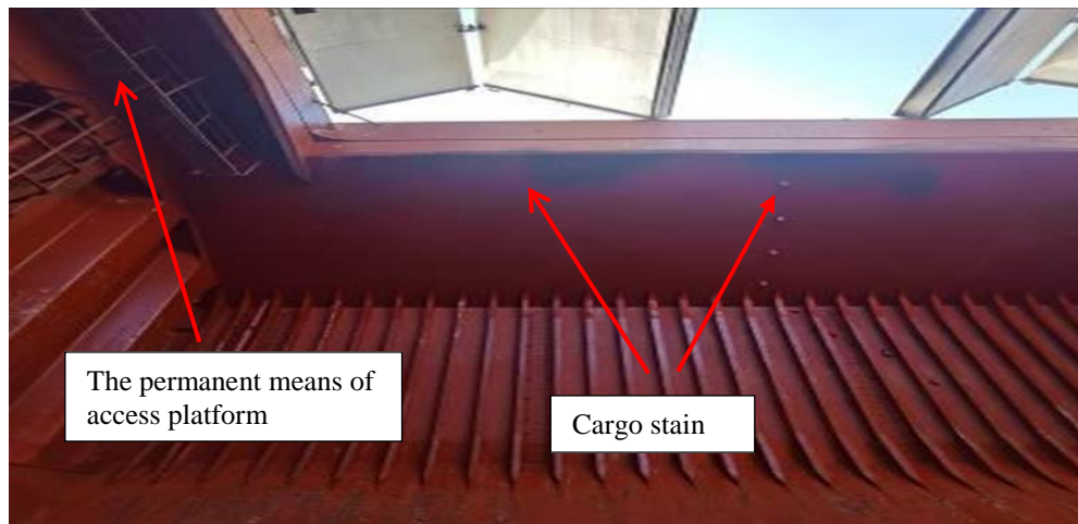
Figure 3 The view of the topside tank bottom of the cargo hold
