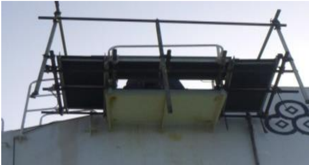
Figure 2 Scaffolding extension rigged to the outboard maintenance platform (Looking Upward)
