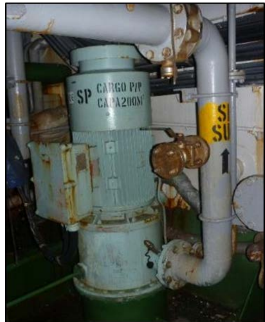
Fig. 20 - Deep well cargo pump on deck
