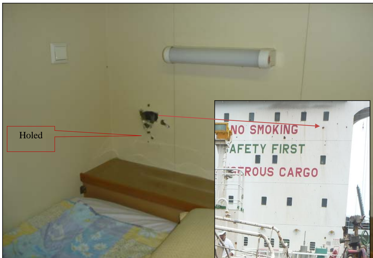
Fig. 7 - Accommodation forward bulkhead in Chief Engineer's Cabin on Captain Deck
