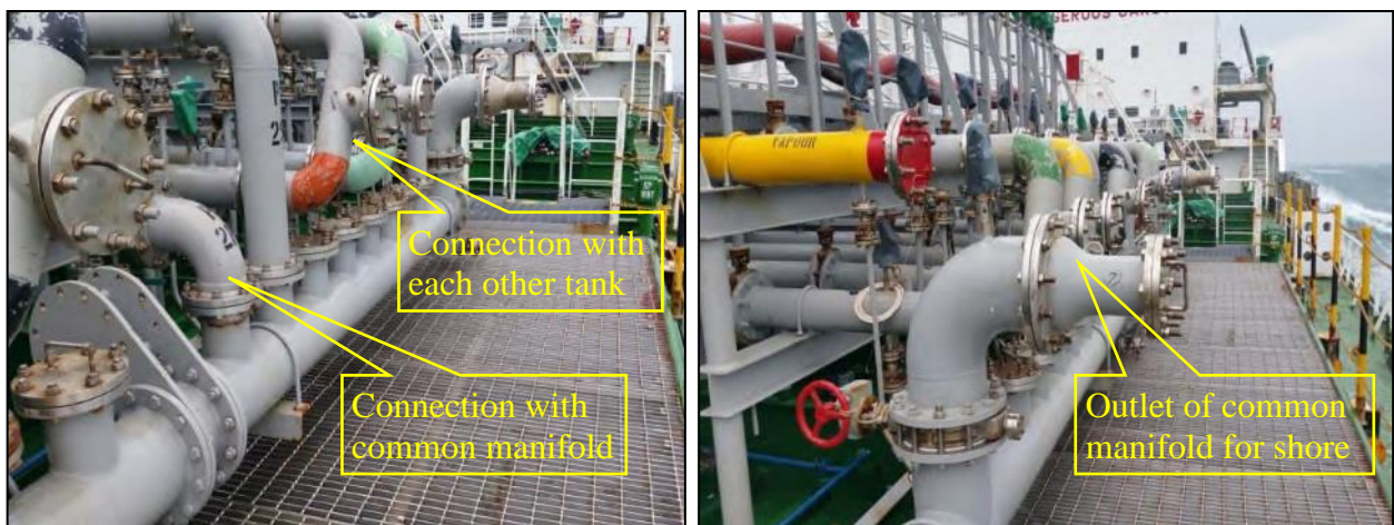
Fig. 16 - Typical connection of manifold by elbow spool pieces
