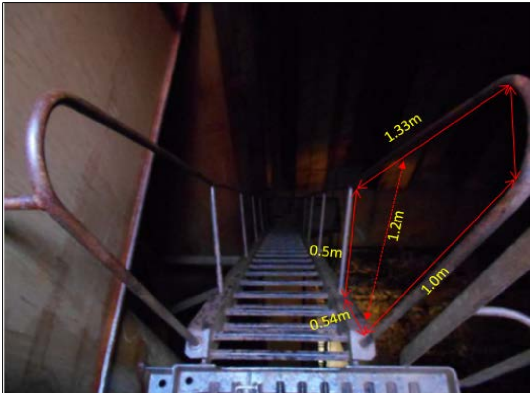
Fig. 6- Photo taken from uppermost platform to show the opening dimensions (i.e. the gap).
