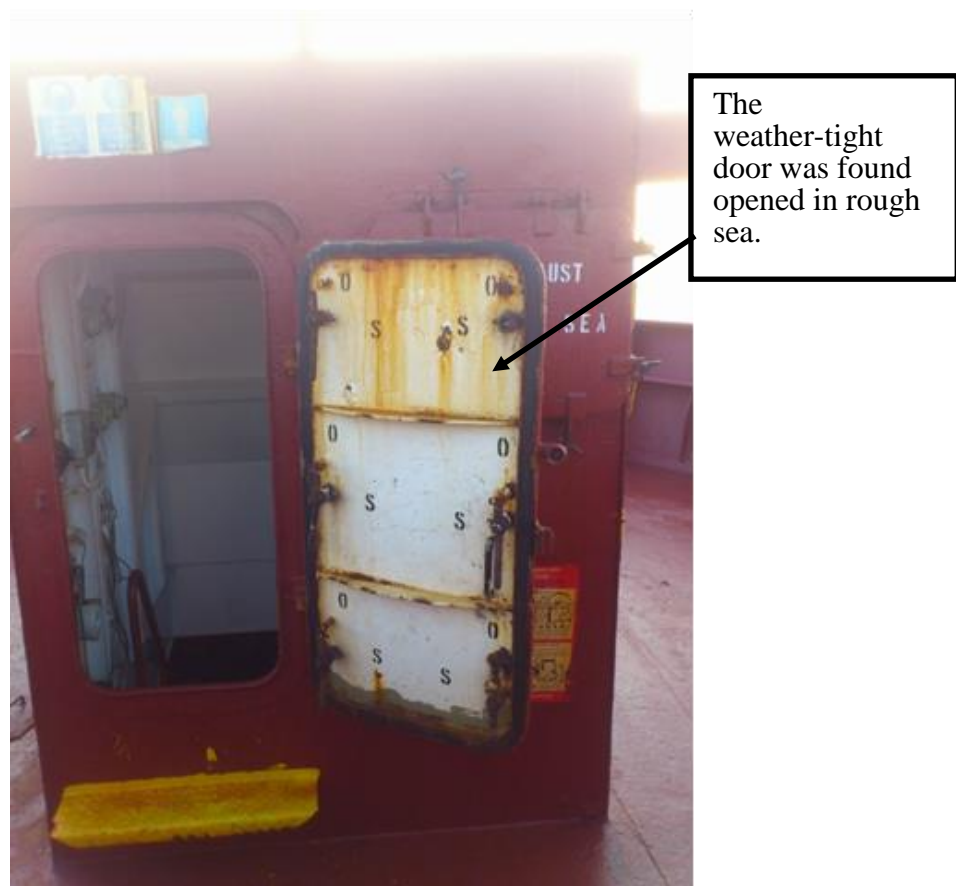
Fig.2 The weather-tight door on the forecastle deck
