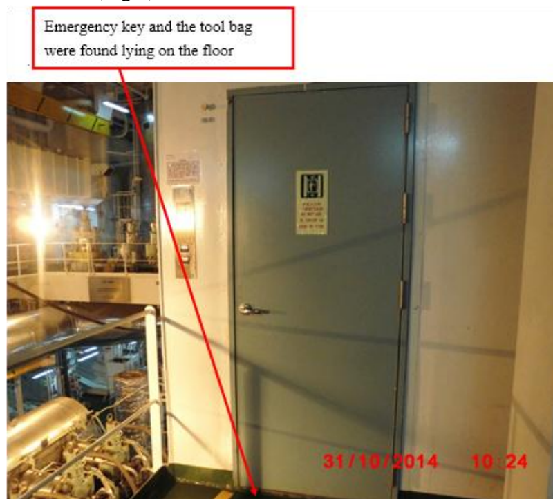
Fig. 2: Elevator Entrance Door at Engine Room Second Deck
