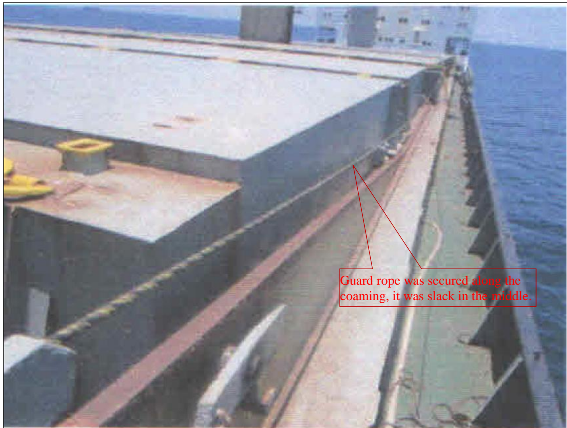
Fig.5 – view from forward, a guard rope was secured along the coaming.
