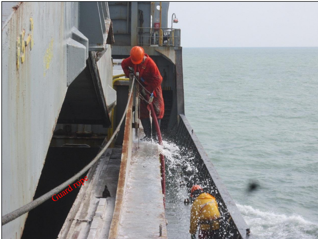
Fig.2 – Arrangement for working on the gutter way of coaming.
