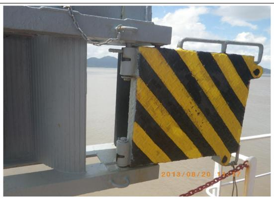
Figure 2: the lower platform at normal secured condition (both locking pins were plugged in)
