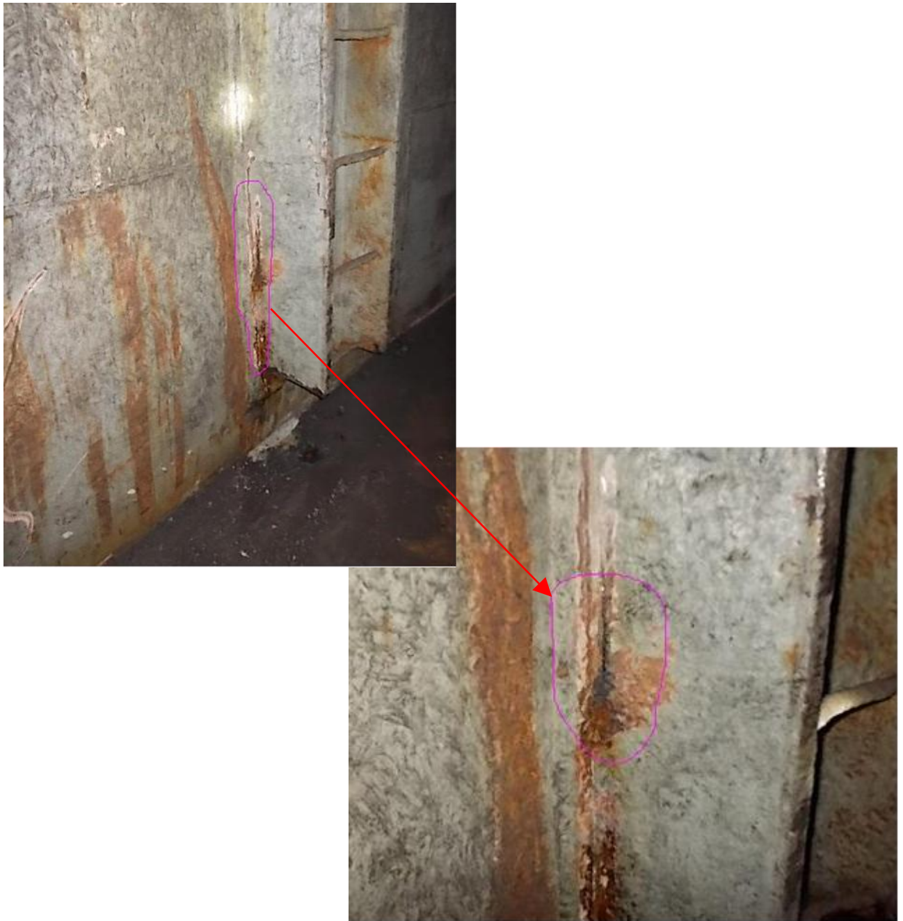
Fig. 4: Suspected area of water seeping out.
