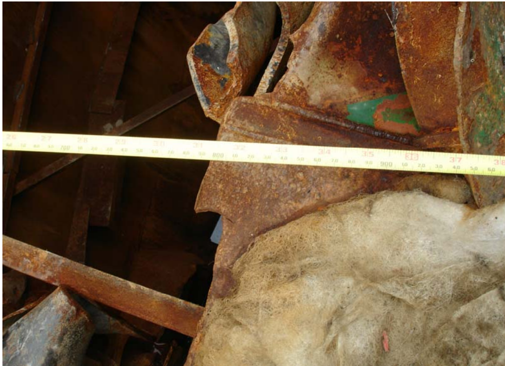
Figure 3 – Maximum inboard collision penetration as measured at open weather deck was about 1 metre
