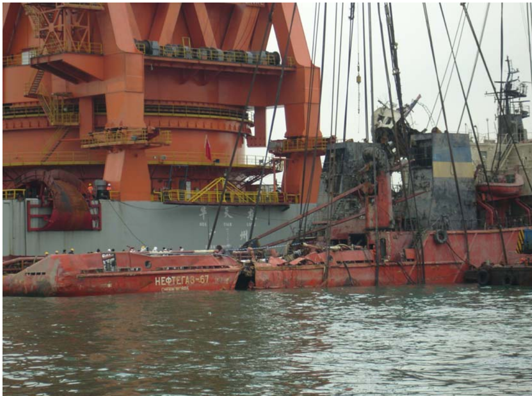
Figure 2A – Damage on starboard side of Neftegaz 67
