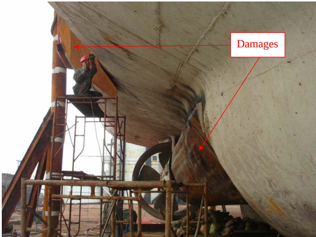
Figure 4 – Damages on starboard side and starboard sterntube of Neftegaz-67
