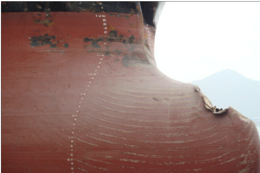
Figure 9- Damage on the bulbous bow of Yao Hai
