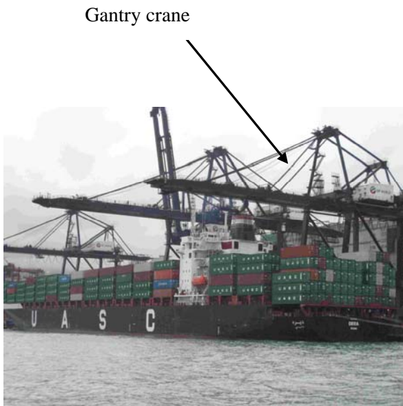
Fig.4: Gantry Crane at the Berth
