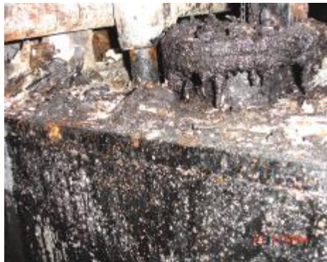
Fig 8: Sign of fuel oil leakage from the top of the boiler fuel oil
