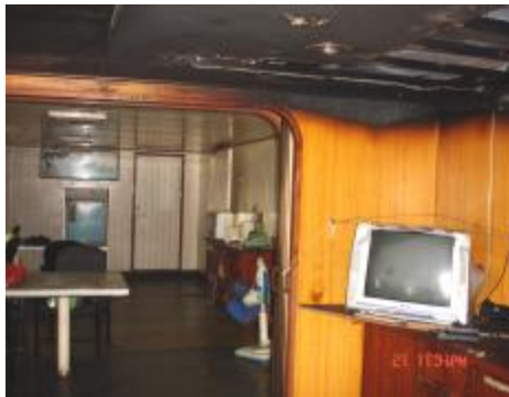
Fig. 15: The roof of the officer's smoking room .
