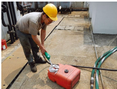
Oil absorbent cotton surrounding the fuel inlet to absorb oil spills
