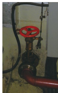
Emergency fuel supply shut-off valve
