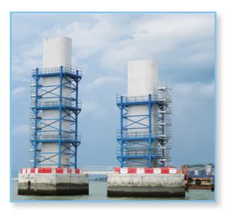
▲ Safety harnesses with continuous and effective anchorage system should be provided when it is impracticable to provide a suitable working platform, access and egress and safe place of work.
