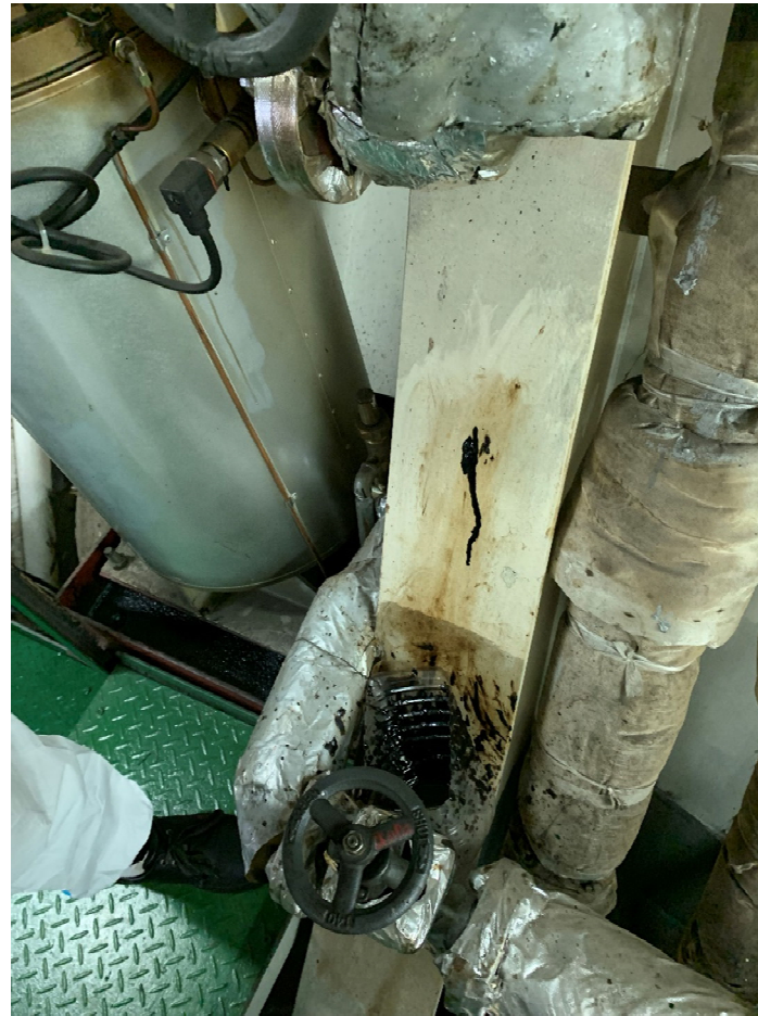
Pipe Condition, leakage and insulation
