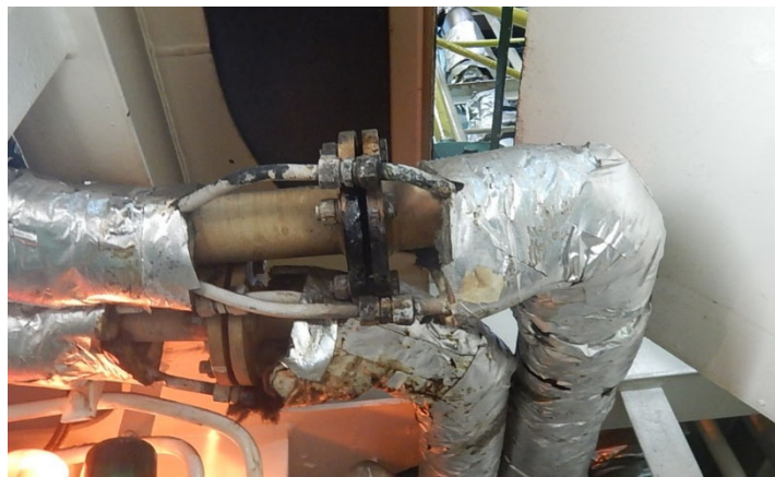
Pipe Condition, leakage and insulation
