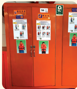
Location 1 : Lifejacket cabinets
