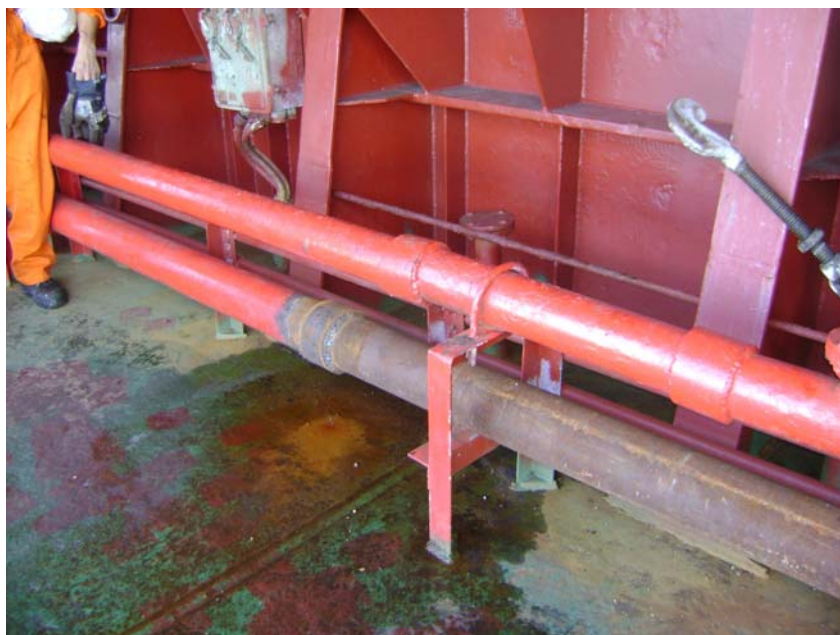
Figure 5 – Deck fire main after repair
