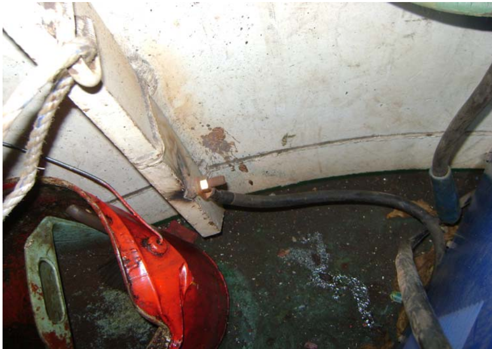
Figure 7 – Fixed welding machine inside No.4 mast house used by Fitter B
