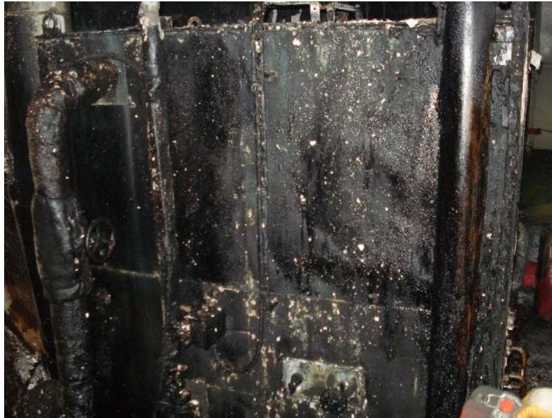
Figure 6: Sign of oil spillage from the blended oil tank.
