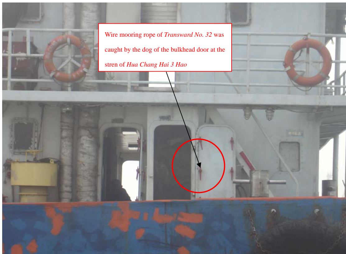
Figure 3 – Diagram showing the dog of the bulkhead door where the wire mooring rope of Transward No. 32 was caught
