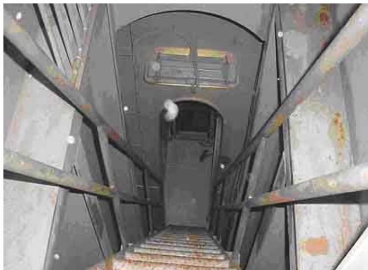
Figure 3: The enclosed stair trunk
