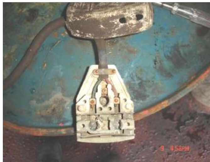
Fig. 6: Internal inspection of the power socket
