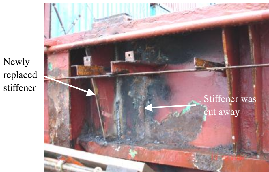
Fig. 2: Repair work on the hatch coaming
