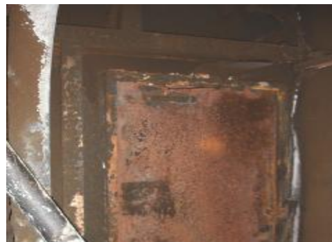
Fig.14: Engine room door at poop deck was badly burnt.
