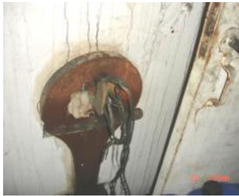
Fig. 21: Ropes used for securing the steering gear room door.
