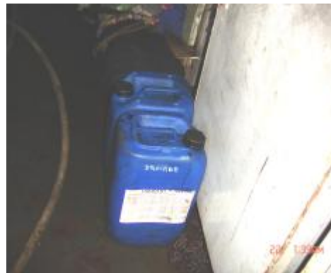
Fig. 22: Drum for keep the steering gear room door open.
