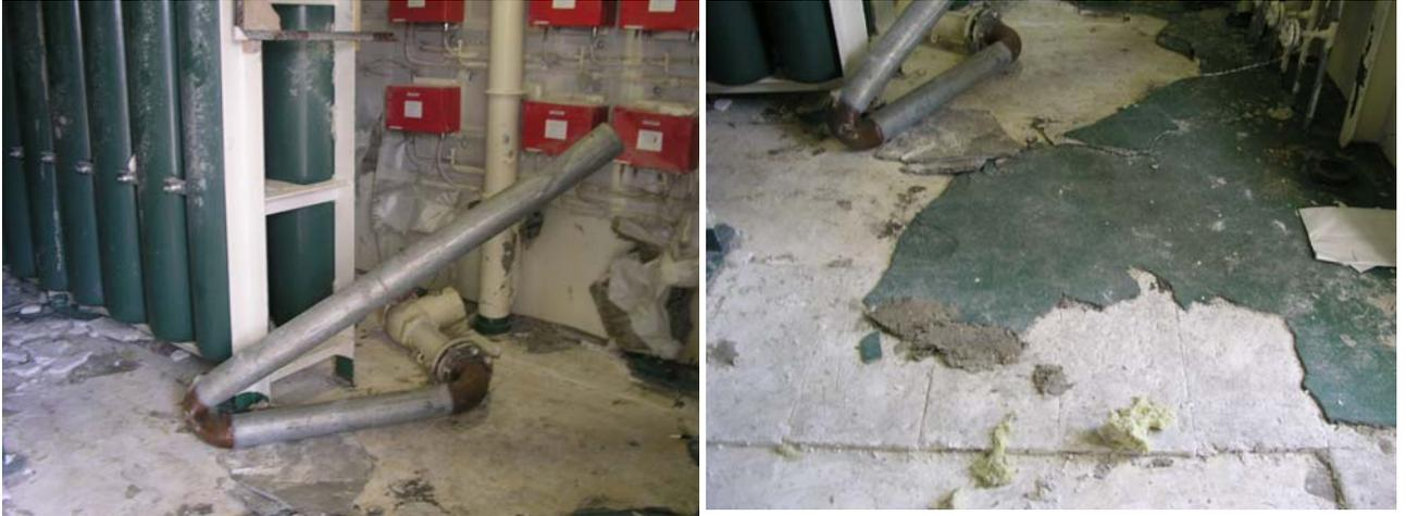
The bended pipe and the damaged floor insulation material after the accident
