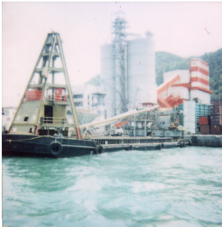
Fig. 2 Sand Barge “永迅” secured to the cement pier
