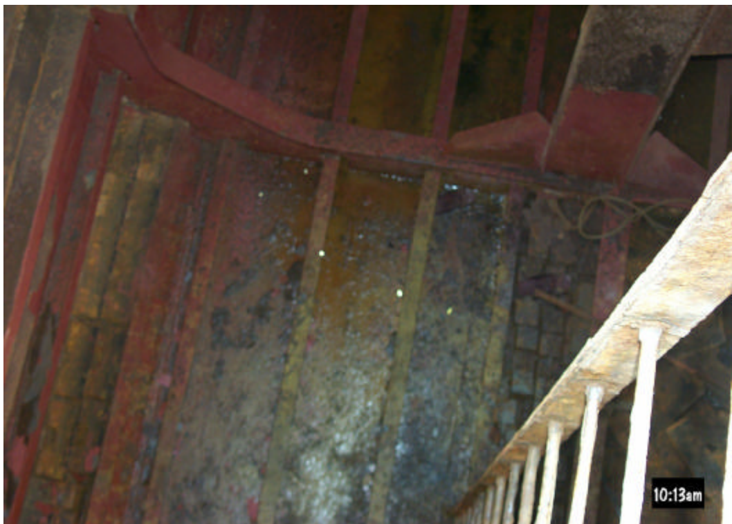
Fig. 2 Internal structure of No. 4 starboard buoyancy chamber
