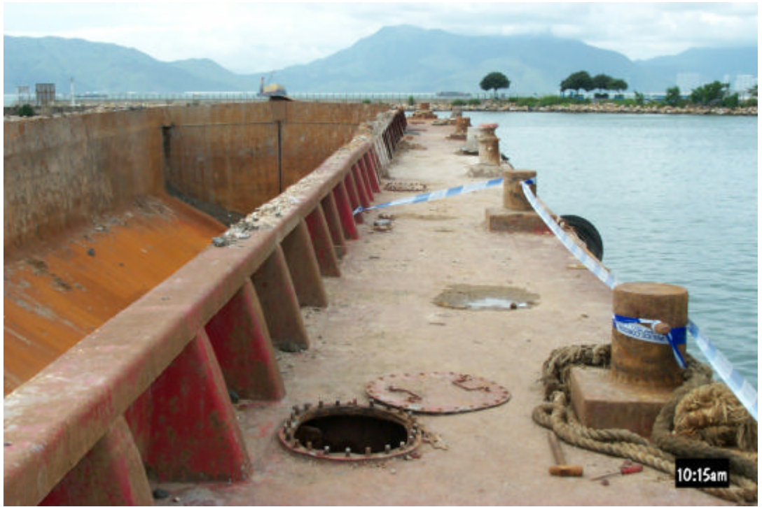
Fig. 1 Location of manhole at No. 4 starboard buoyancy chamber
